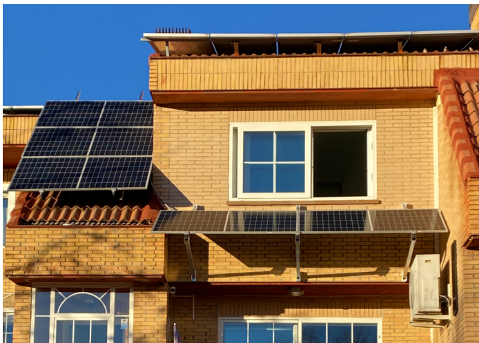
The front of the house includes solar modules on any available roof-space and a solar awning
