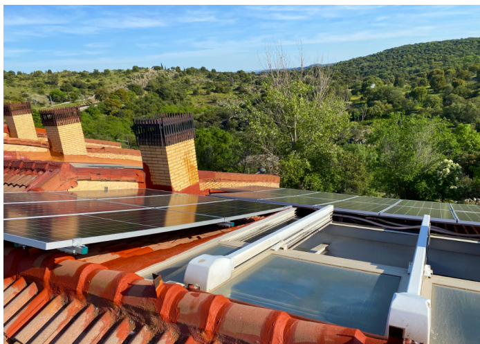
The southern pitch of the roof features 20 modules surrounding a wide skylight and two big chimneys
